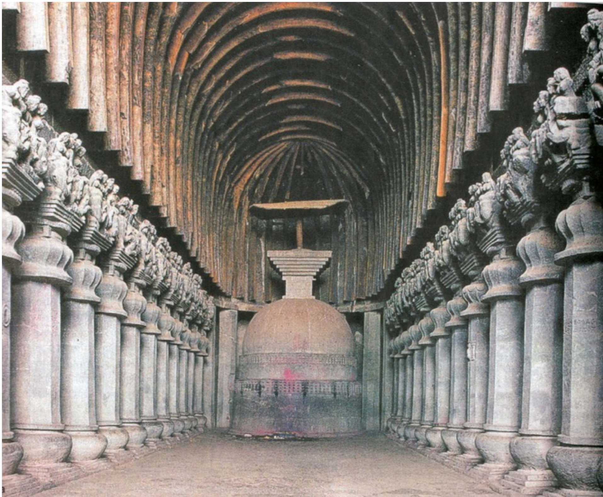
Karla cave prayer hall - Buddhist // Gupta ( 120 CE) (note false ribbed structure of wood)
