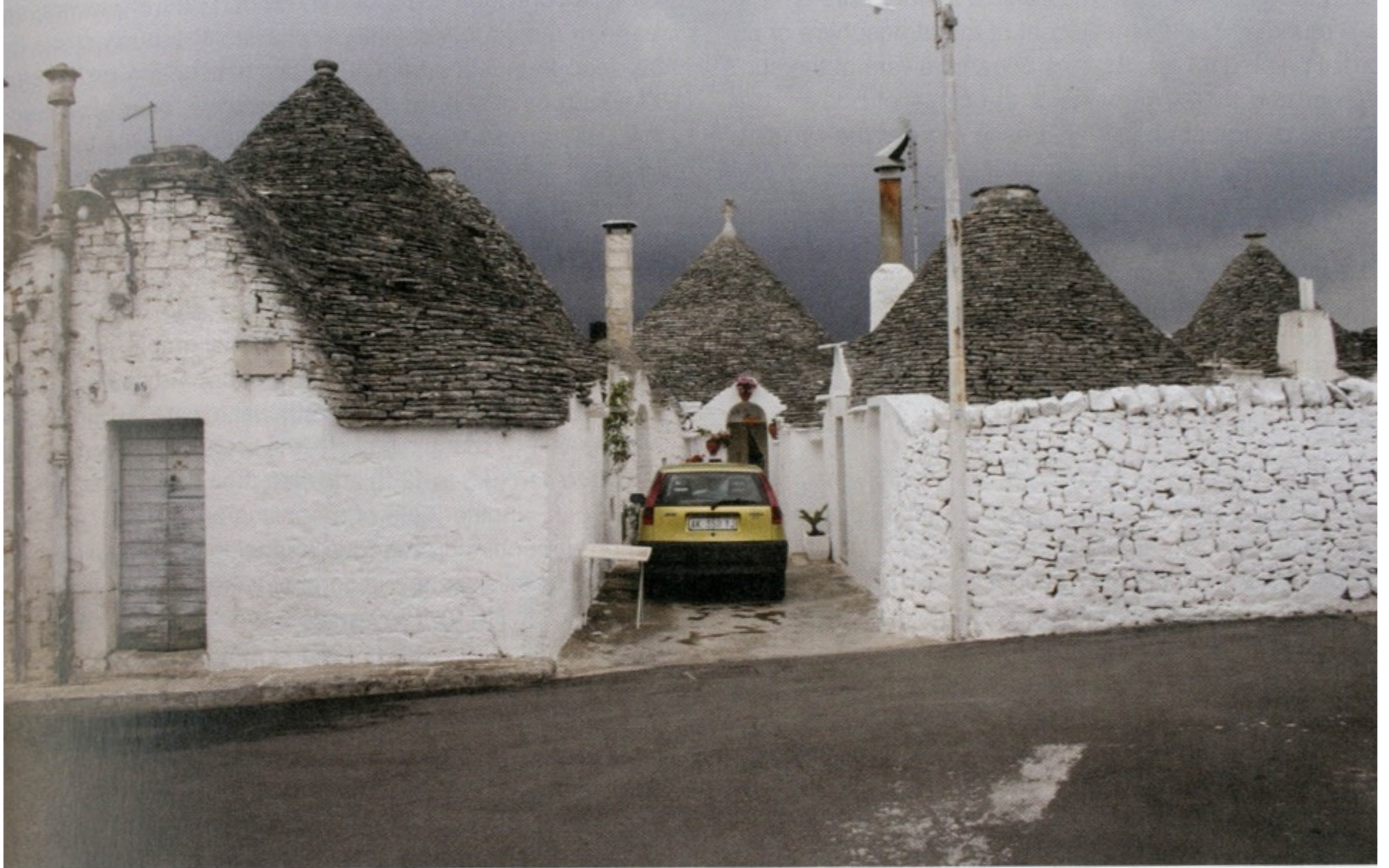
Figure 1.2-10 Alberobello, Puglia, Italy. Row of cone-shaped stone houses built with corbel dome roofs. Cone structures in the region date back to Neolithic times, but most trulli were constructed between 1500 and 1900.
