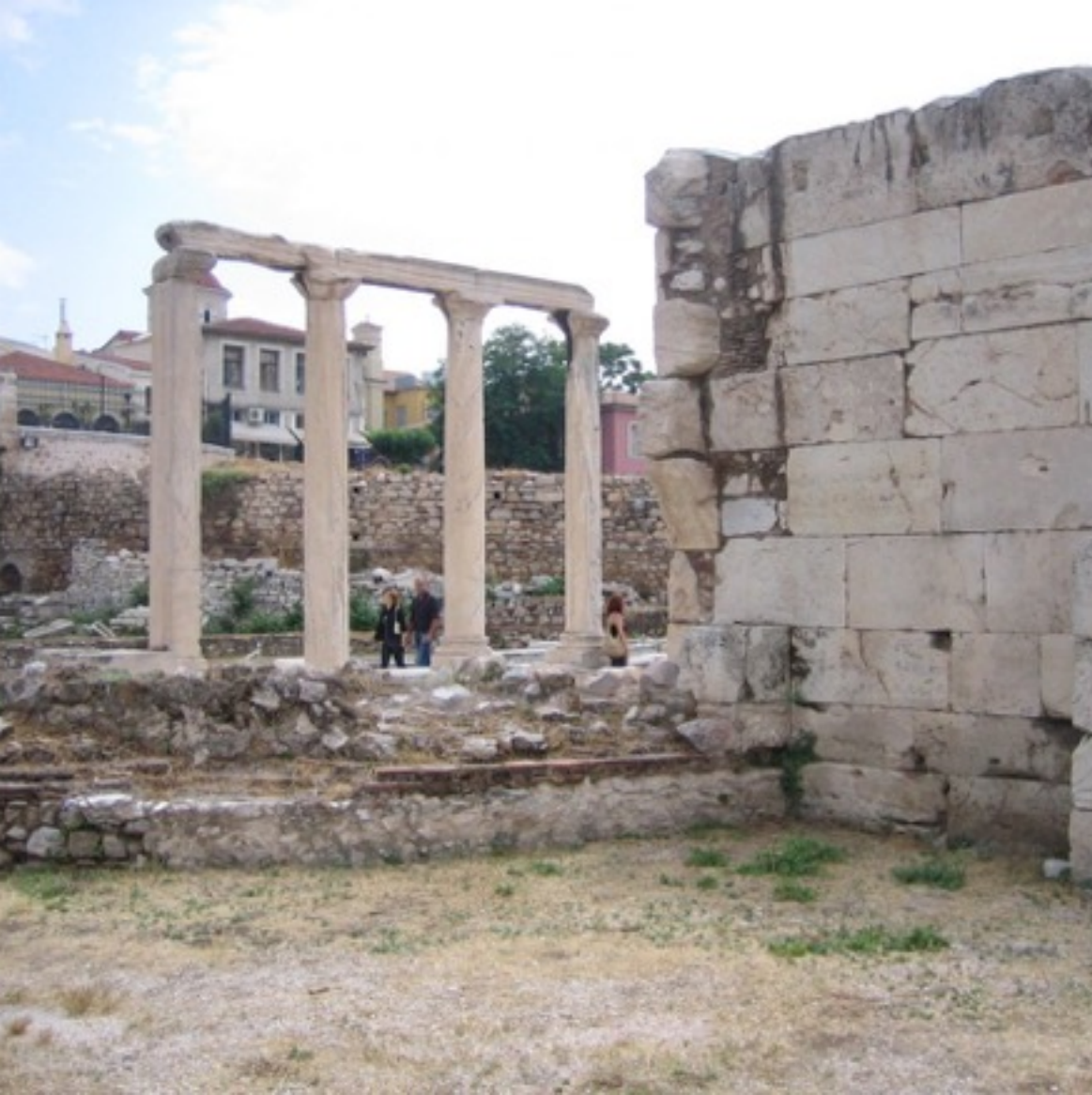
Columns holding up a large beam or lintel ( post & beam or post & lintel )
