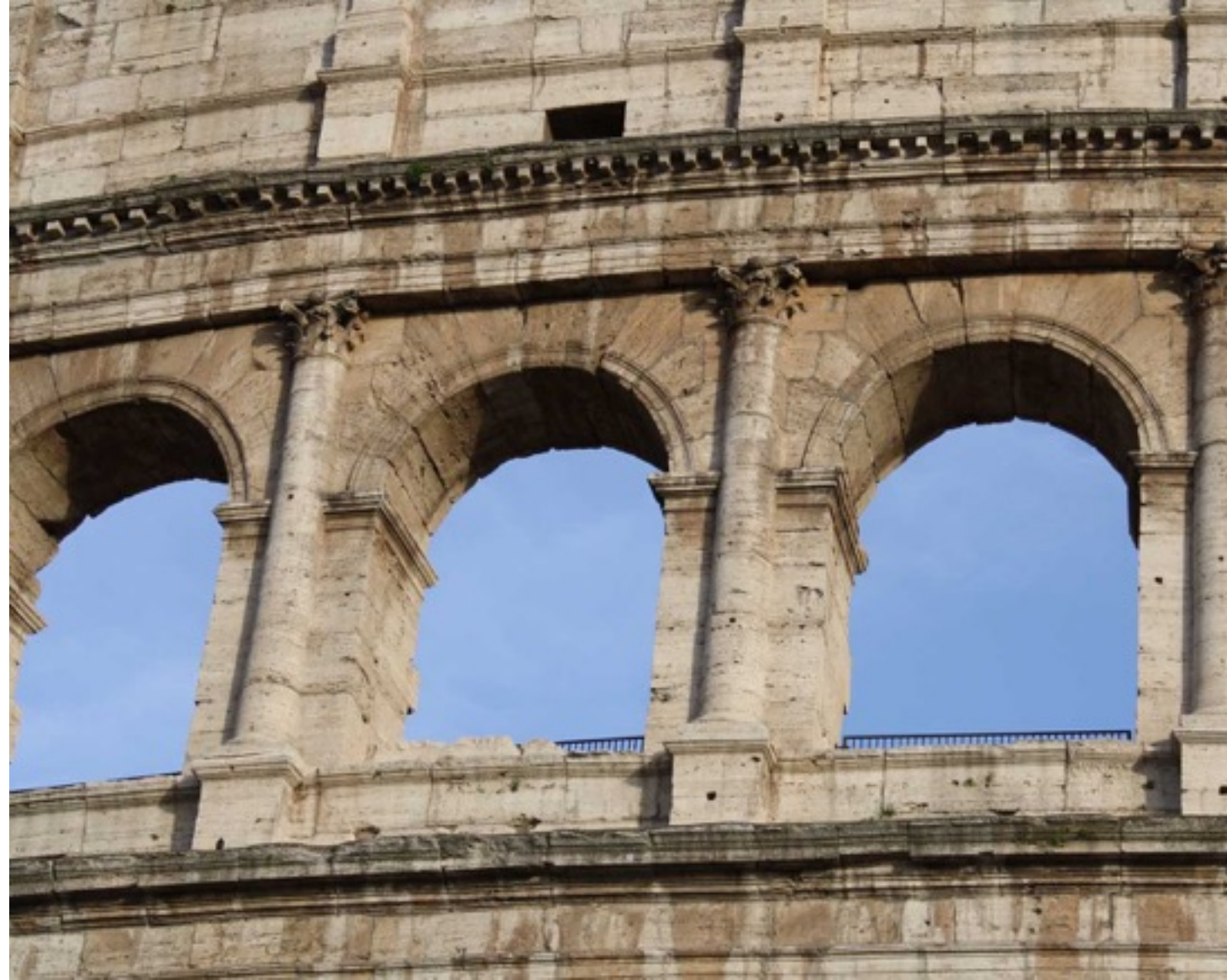
Wall w/ large arched openings and columns (posts) and lintels applied to it
