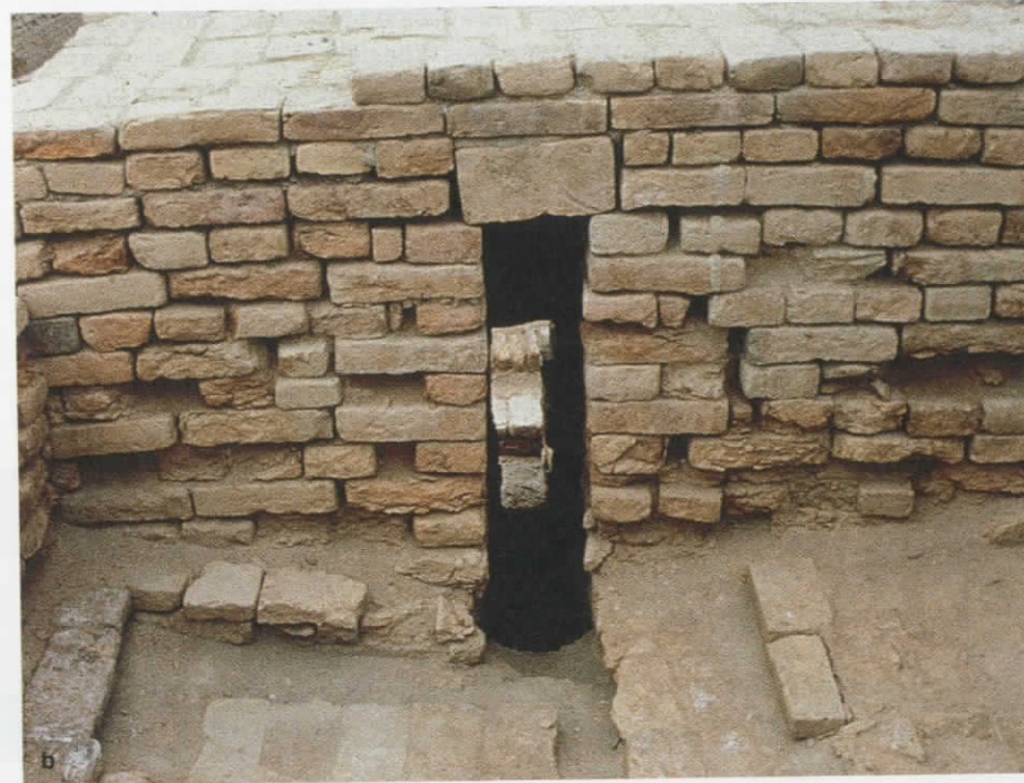
Figure 2.3-1 (a) The Indus valley region. The Saraswati (now Ghaggar) River changed course in the second millennium. Harappa can be seen in the north, Mohenjo-daro in the south, and Lothal on the southern coast at the Gulf of Cambay. (b) Mohenjo-daro. Detail of brickwork and drainage at the Great Bath, ca. 2500 BCE.
