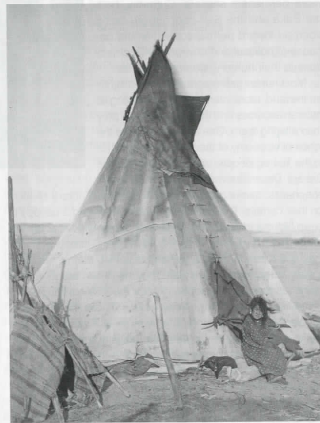
Figure 1.2-2 Pine Ridge reservation, Dakota territories. Sioux tipi photographed by John Grabill in 1891, showing canvas flaps for chimney and entry.
