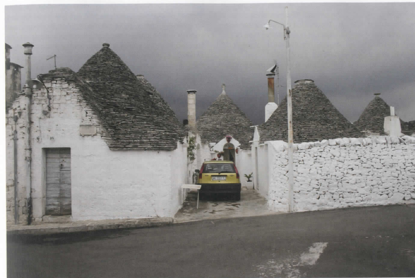
Figure 1.2-10 Alberobello, Puglia, Italy. Row of cone-shaped stone houses built with corbel dome roofs. Cone structures in the region date back to Neolithic times, but most trulli were constructed between 1500 and 1900.
